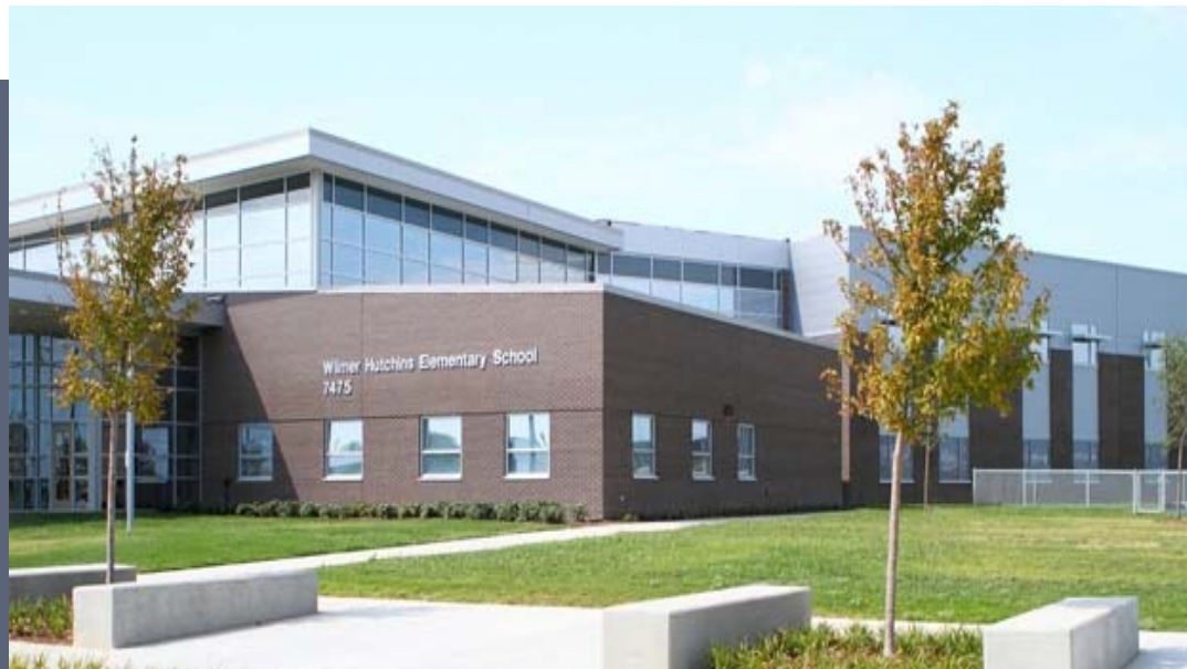
Wilmer Hutchins Elementary School: A Dallas Independent School District Campus
